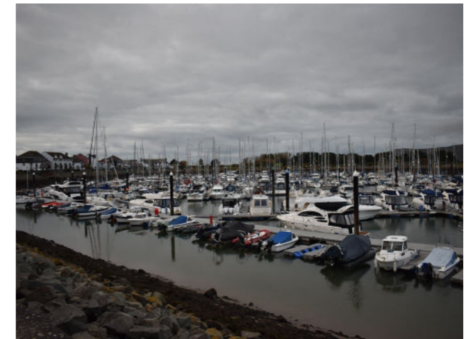
Figure 43A and 43B, Conwy Marina showing the rock surrounding rather than a solid marina wall © Conwy Marina
