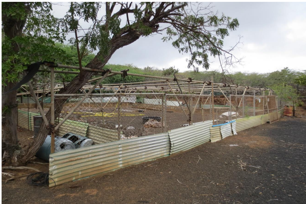
Figure 2: The remains of the shade greenhouse (photographed August 2018) previously used by the Ascension Island Gardeners Club. The shade netting has rotted away, but the structure looks sound.
